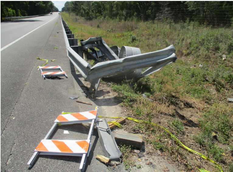
FIGURE 2- Crushed guard rail, at a site of an accident, near Rice Creek
